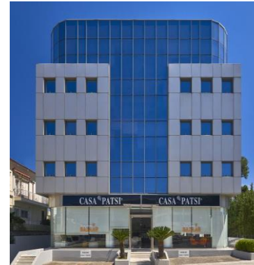
Mesageion Ave. Office Building
