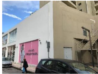
Outdoor Stair to Mezzanine
