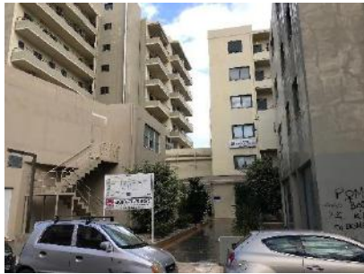
Access to Mezzanine
